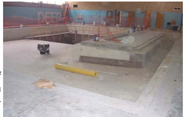
New Pool Ramp and Resurfacing
