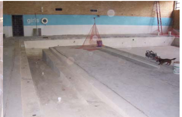
New Pool Ramp and Resurfacing
