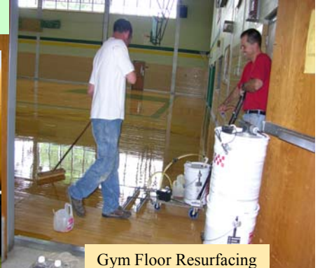
Gym Floor Resurfacing
